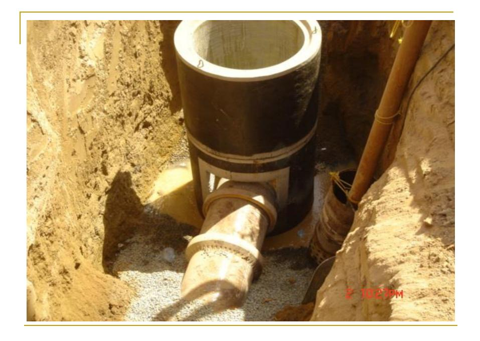
Pushing the pipes together with the crane bucket and a belt.(≥ DN 400)
