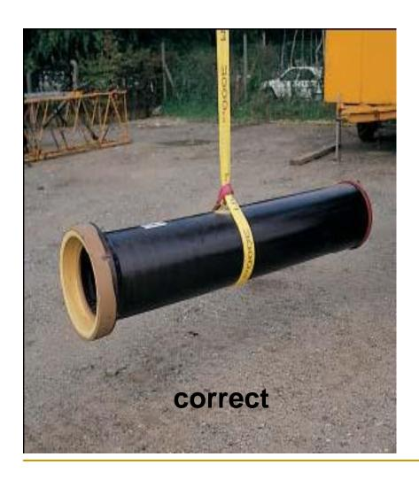
Transport individual pipes with belts (mark on crown – yellow or white spot = centre of gravity – pipe hangs level).
