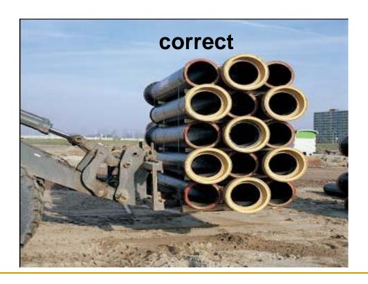
When placing the pallets longitudinally on the forks, place protective timber between the parcel and the fork's base. Better is to transport the parcel in transversal direction on the fork teeth.
