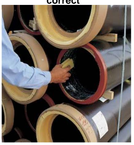
Before the pipes are laid, check both ends of each pipe optically and internally with the aid of talcum powder in order to find any cracks that might have occurred in the course of transport.
